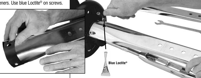
Fasten second long link plate to drum assembly and secure to toggle using locknuts.
